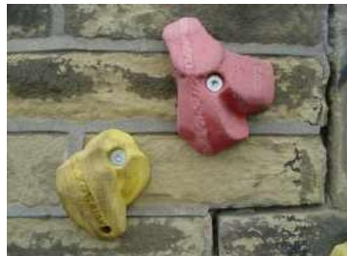
Handgrips need regular monitoring and tightening. They can work loose in the first few weeks after installation. You will receive a specialist Allen key with your installation to tighten the grips.
